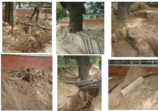
Construction activities around tree basins
