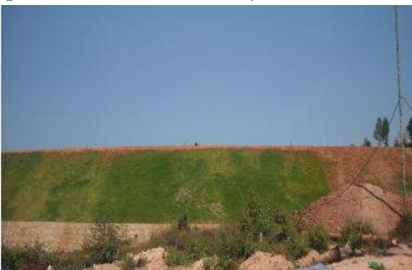
stadium, Kerala. b) Comparison of growth of seeded Bermuda grass at the stadium with and without the use of geotextiles.
