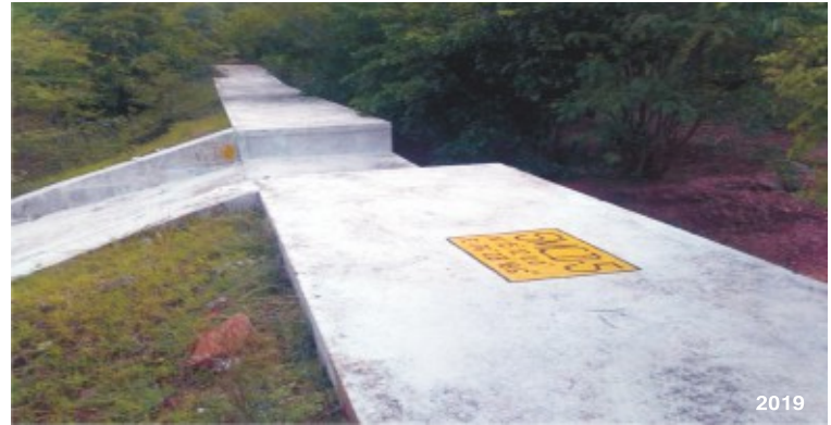
Stone Masonry Check Dam
