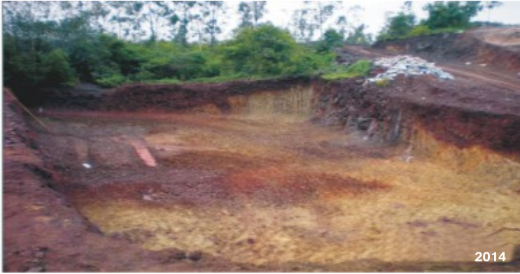
Silt Settling Tank
